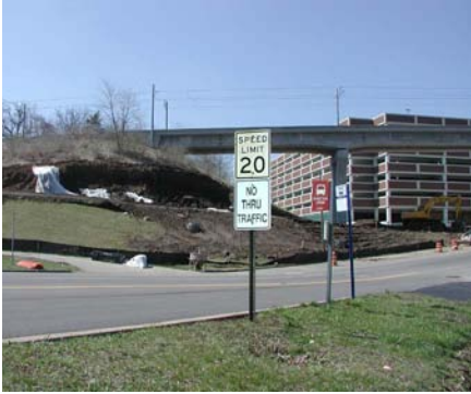
Construction of TrailNet pathway in 2005.
